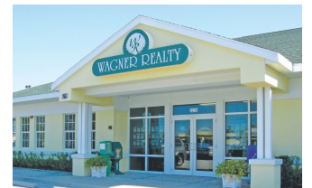
5215 SR 64 East Bradenton, Florida
